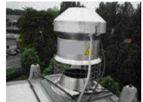
Optimised shape to enhance the impact of wind on extraction flow
