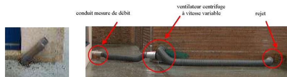
Mechanical extraction from the void
