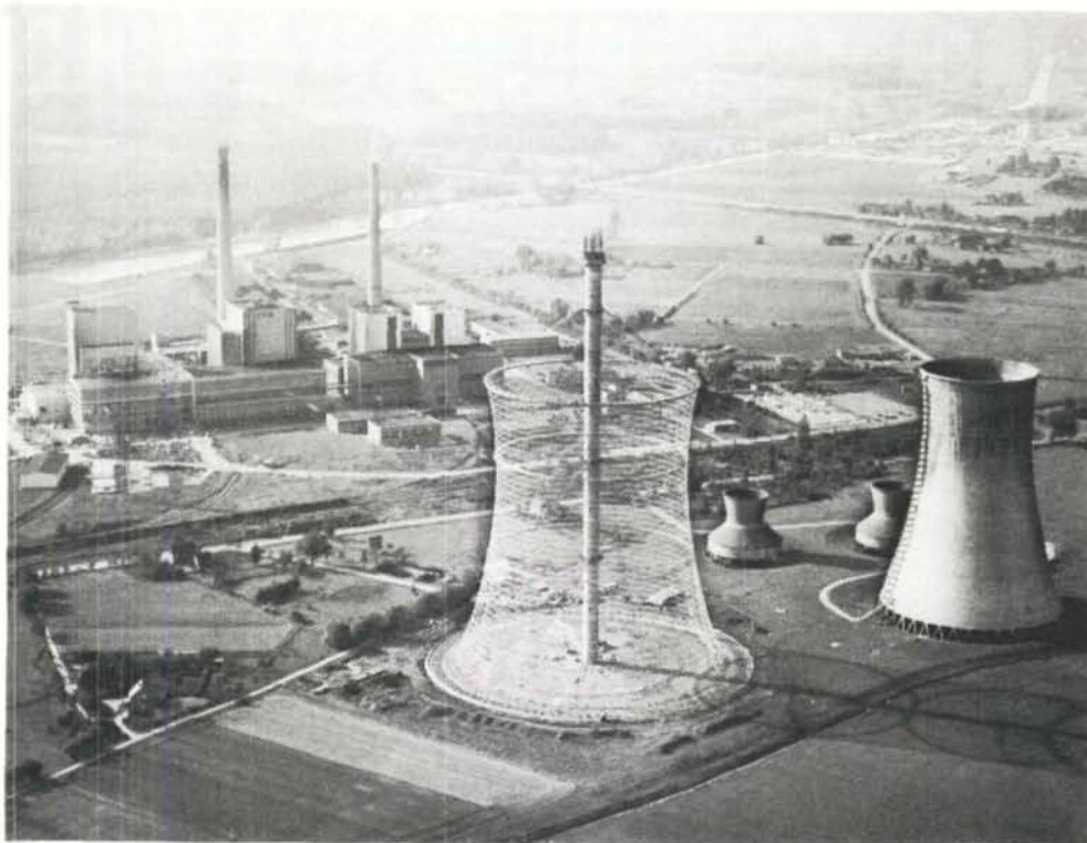
The thorium high temperature reactor under construction at Uentrup, Fed.Rep. of Germany, is connected with currently operating fossil power plants. In the foreground a dry cooling tower under construction. Photo: VEW
