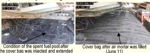
Condition of the spent fuel pool after the cover bag was injected and extended (June 8)
