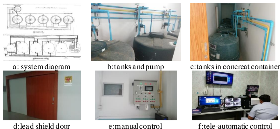
FIG. 1. Showing the semi- automatic I-131 waste management system.
