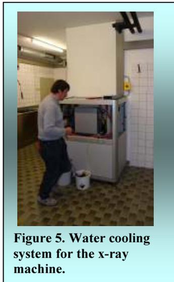
**Figure 5. Water cooling system for the x-ray machine.**
