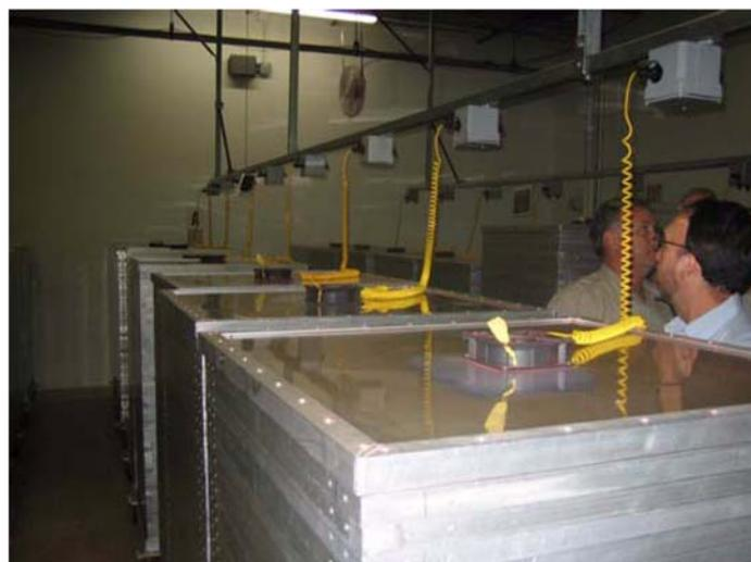
**FIGURE 2: The voltage of fan systems on towers requires monitoring (L12). Towers with fans are unsuitable where electricity is costly or unreliable; or if emergency generators are unavailable**
