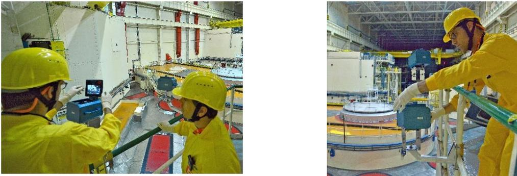
Figure 1: New IAEA Safeguards inspectors are being trained to install and adjust XCAMs, the new generation surveillance cameras at the Dukovany Nuclear Power Station (Czech Republic).
