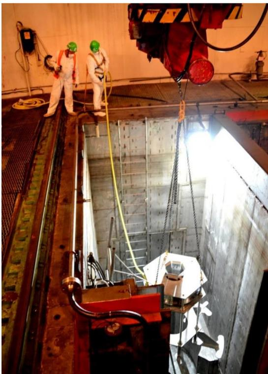
Figure 2: Installation PGET for VVER-1000 measurements at Balakovo NPP.
