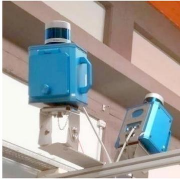
Figure 2: LIDAR-based Laser Curtain for Containment (LCCT) System installed at a safeguarded facility.
