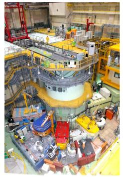
HANARO complex is composed of the HANARO research reactor and ancillary facilities such as the Cold Neutron Research Facility (CNRF), Radioisotope Production Facility (RIPF), and Irradiated Material Examination Facility (IMEF). The HANARO and ancillary facilities were designated as an ICERR by the IAEA in 2019.
