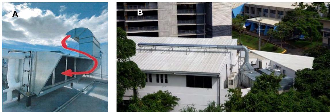
**FIG. 1.** A. Inlet and outlet pipe HVAC system initial arrangement installed in the building and radioactive gas trajectory entering production main floor. B. Final placement of the outlet pipe.
