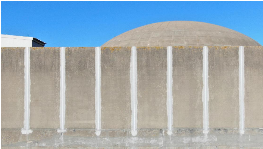
Monitoring of the dike
