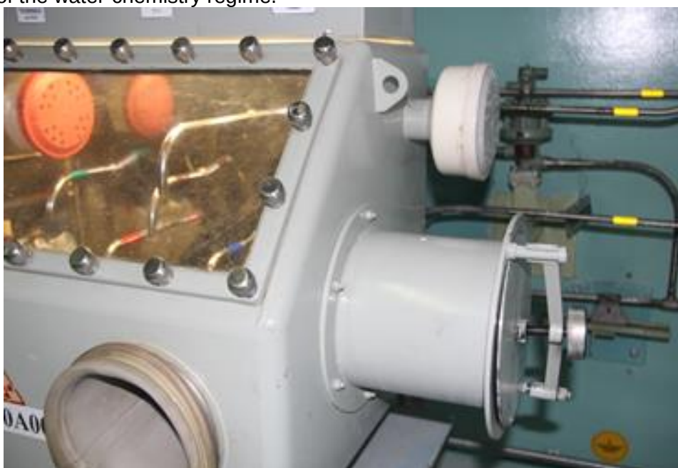
Sampling box (before modification by the plant): O 2 /H 2 manual measurement
