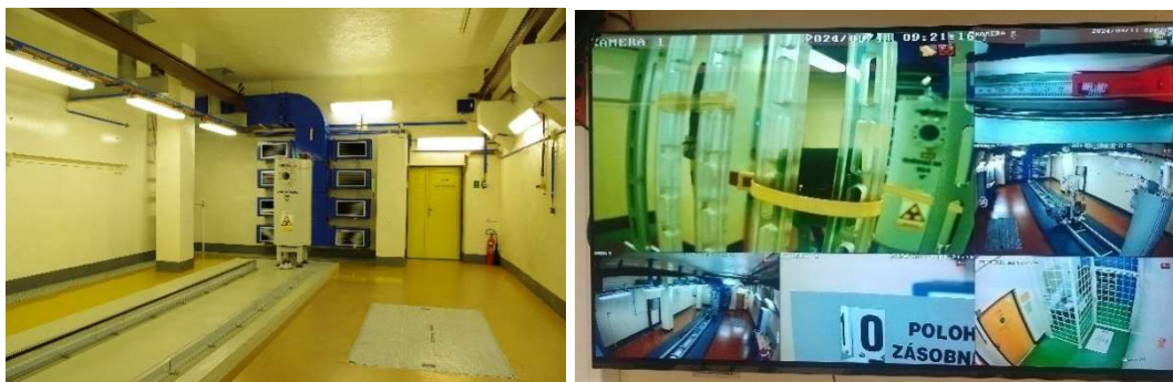
Remote view of calibration area from control room
