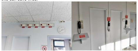
Differential pressure gauge indicating the pressure difference between inner and outer spaces mounted on the entrance door.
