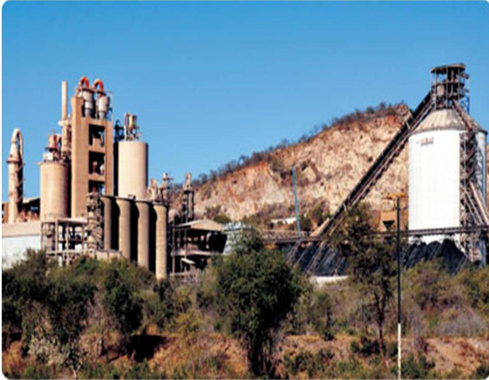
Grinding consumes 1/3 of the power required to produce 1 ton cement, 30-40 kWh/ton
