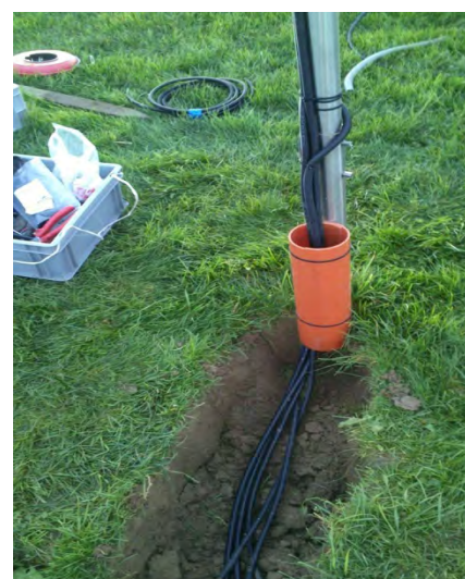
FIG. 4: Protecting data network cables at the Grabenegg experimental station
