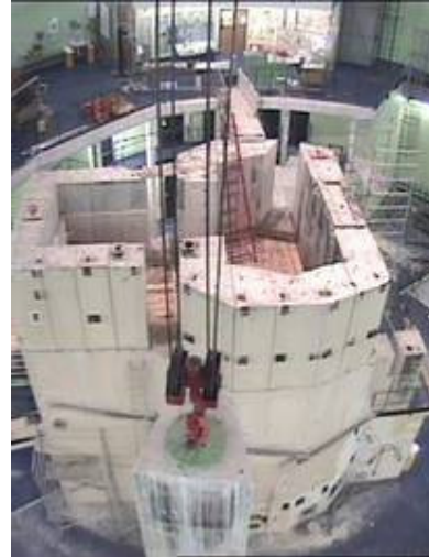
Dismantling of the biological shield: Layers designated for cutting Removing of blocks
