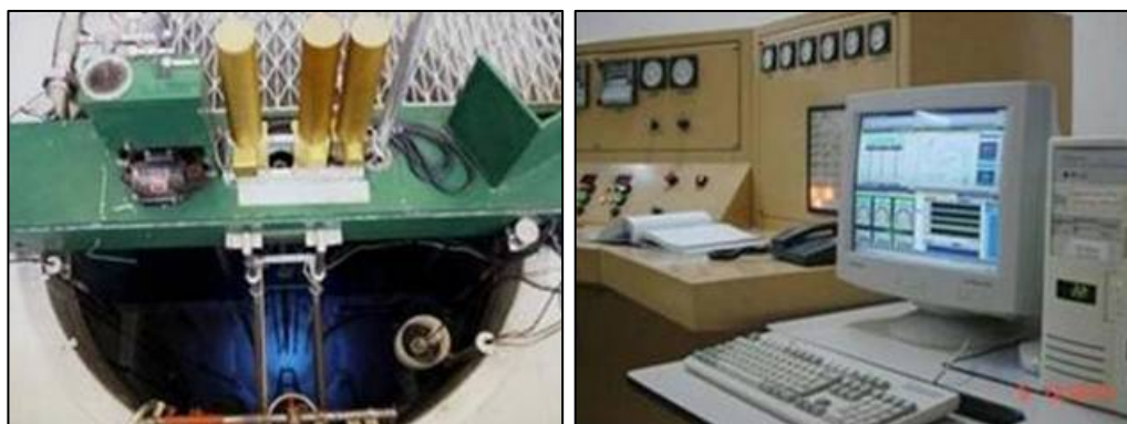
Figure A.2. IPR-R1 – Reactor Core and Control Room
