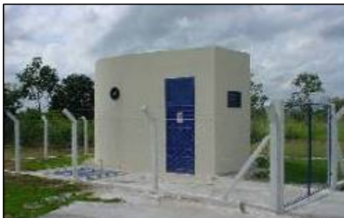
Figure D.2. Interim storage facility at CRCN-CO
