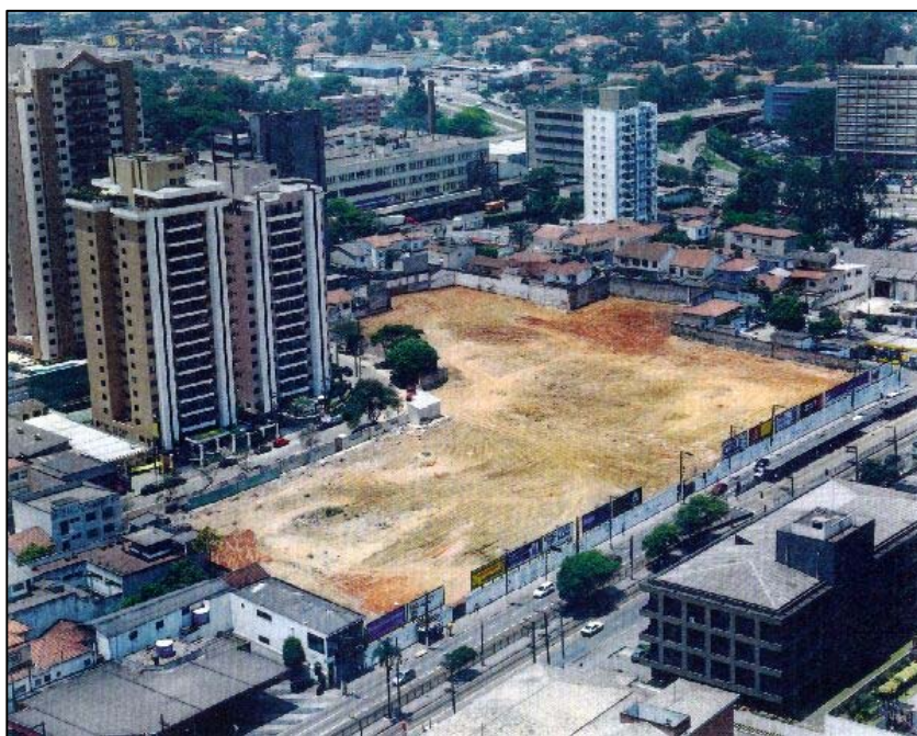
Figure F.10. Clean area after USAM decommissioning work
