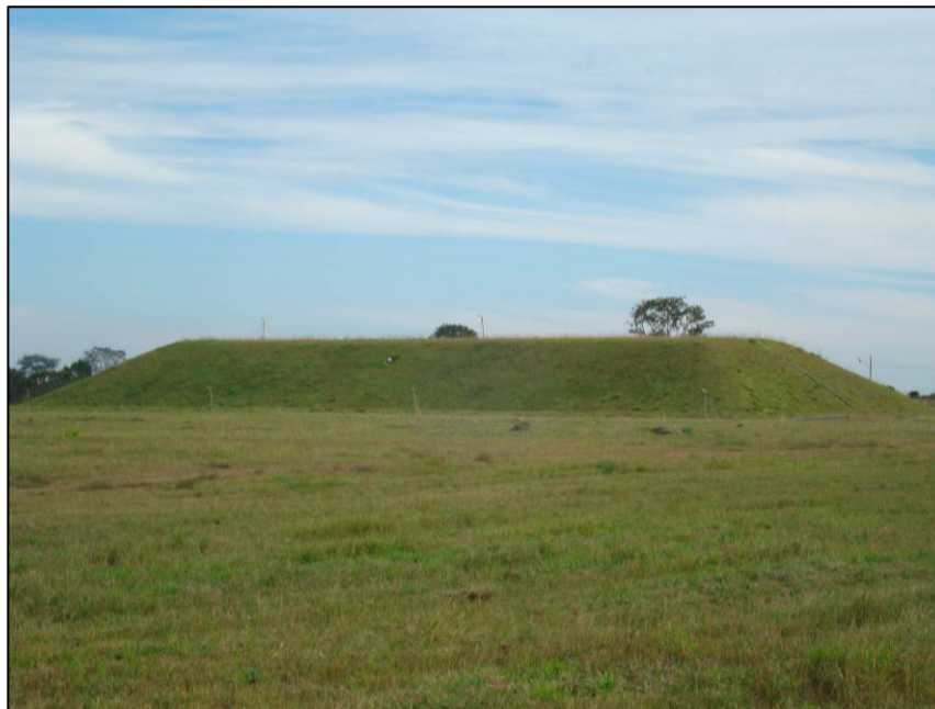
Figure D.5. Repository at Abadia de Goiás
