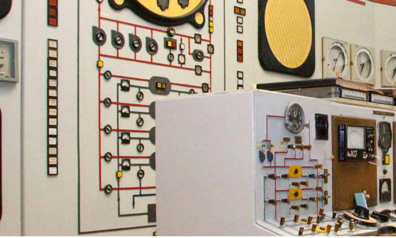
The name AM-1 is derived from the Russian phrase Атом Мирный, pronounced 'Atom Mirny'or 'Peaceful Atom'. Its reactor, which was controlled from the main control room, had a net capacity of 5 MW. In this photo, the operator is monitoring the status of the 18 fuel rods.
