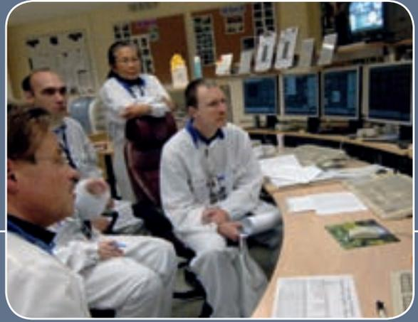
**4** Inside a control room, inspectors eye screens displaying schematics of the plant's operational flow. Computer programs monitor key operations — temperatures in the pipes, conductivity measurements, batch weights, precipitation levels, Ph balance and chemical flows, among others. Closed circuit TV cameras zoom in on gauges giving the operator critical indicators from the control room.
