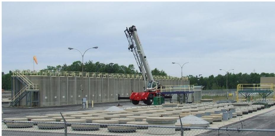
**Figure 5.33: Schematic of in-ground storage structures at Western WMF (note: only 2 of 6 resin liners are shown)**
