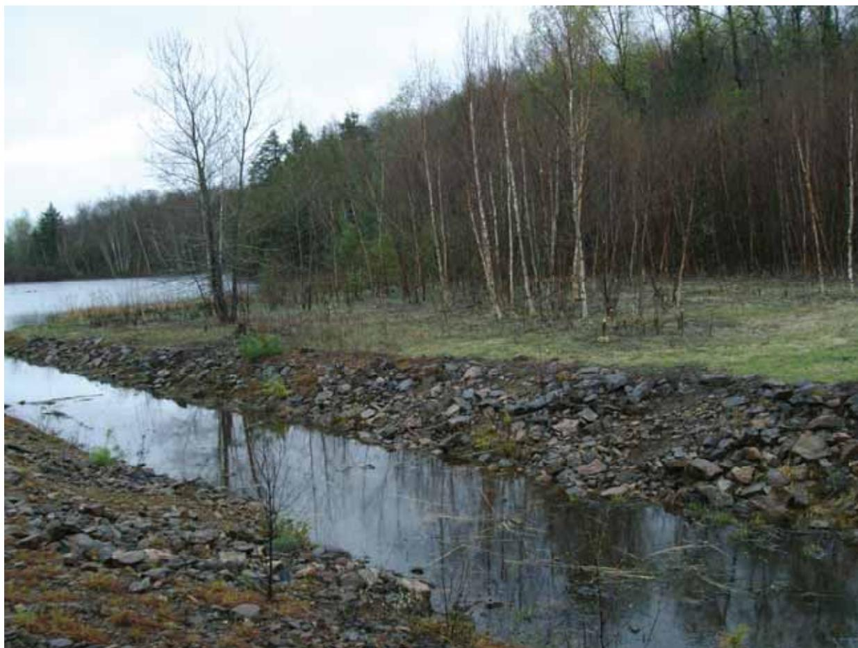
**Figure 8.8** – South tailings basin spillway at Bicroft Tailing Storage Facility
