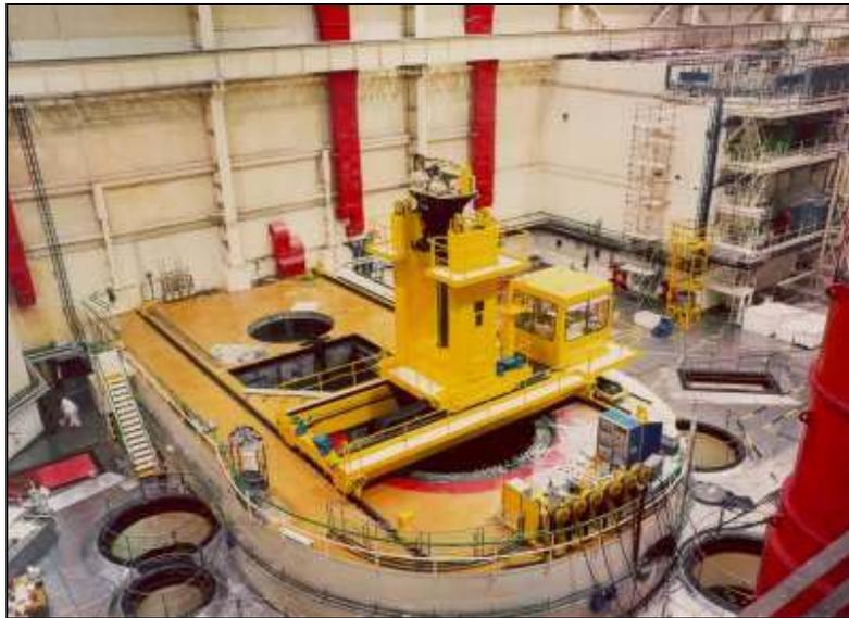
Fig. 4.1 Uncovered SF pool and ŠTK during reactor refueling
