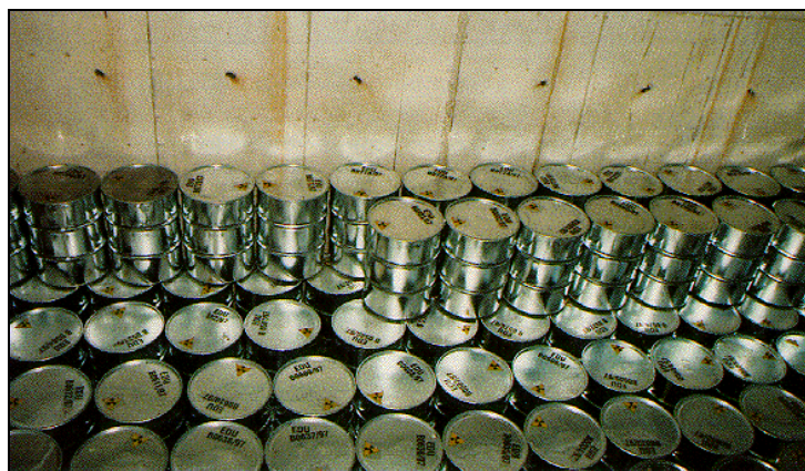
Fig. 8.4 View of partly filled vault in RAW repository Dukovany
