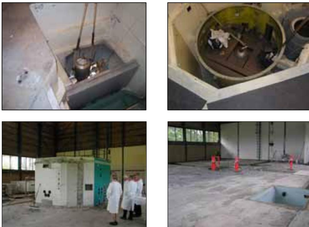
Figure 2. (Upper left) removal of the recombiner, (upper right) removal of graphite and the reactor core, (lower left) biological shield after removal of control rod housing, (lower right) biological shield removed.
