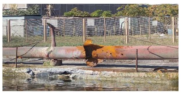
Broken pipe observed by the IAEA staff at the ZNPP site due to shelling on 21 September 2022. (Photo: IAEA)
