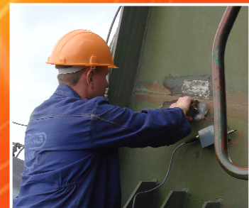
Installing an acoustic emission sensor.
