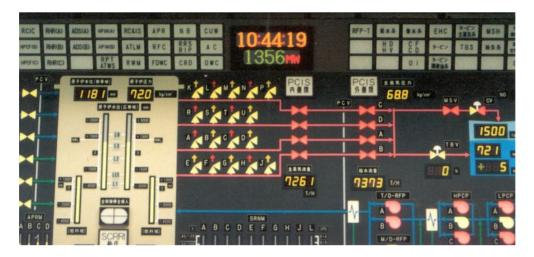
FIG. V-1. Section of main control panel in the Kashiwazaki-Kariwa-6 and -7 Advanced Boiling Water Reactor (1350 MW(e)).
