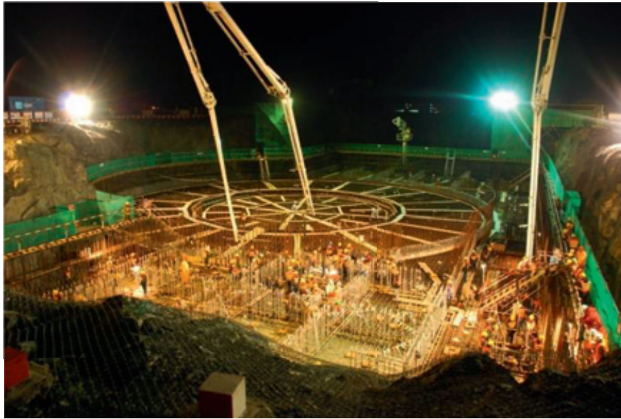
FIG. 1. Pouring the first concrete at the Sanmen nuclear power project site in China.
