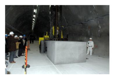
FIG. A-13. Emplacement of the first waste disposal package at the disposal facility in Bátaapáti, Hungary.
