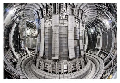
FIG.B-3. The inside of the JET vacuum vessel with the installation of the ITER-like wall completed.
