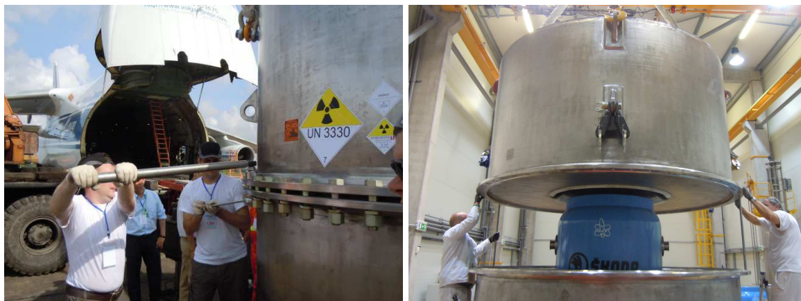
FIG. C-5. Left: Tightening the bolts on special transport packages carrying spent HEU fuel from Viet Nam's Dalat Nuclear Research Institute to the Russian Federation. Right: Placing a protective overpack on a transport cask containing spent HEU fuel from the BRR in Hungary. This overpack was designed to permit air transport.
