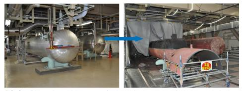
FIG. C.2. Dismantling a high-pressure feedwater heater as part of the decommissioning of the Monju reactor. (Source: JAEA)
