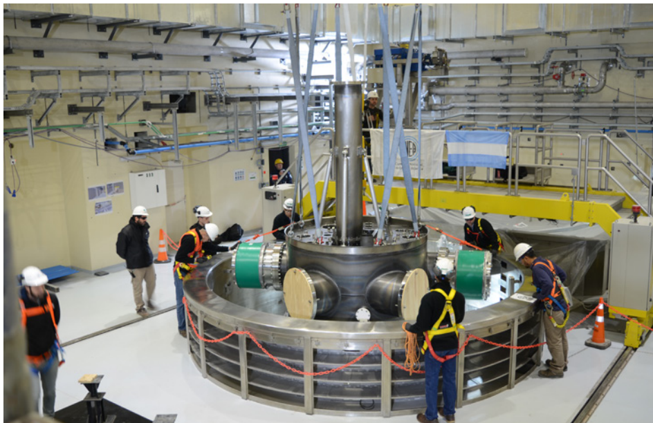
FIG. E.1. Installation of the reflector tank at the RA-10 research reactor, Ezeiza Atomic Centre, Argentina. (Source: National Atomic Energy Commission (CNEA), Argentina)
