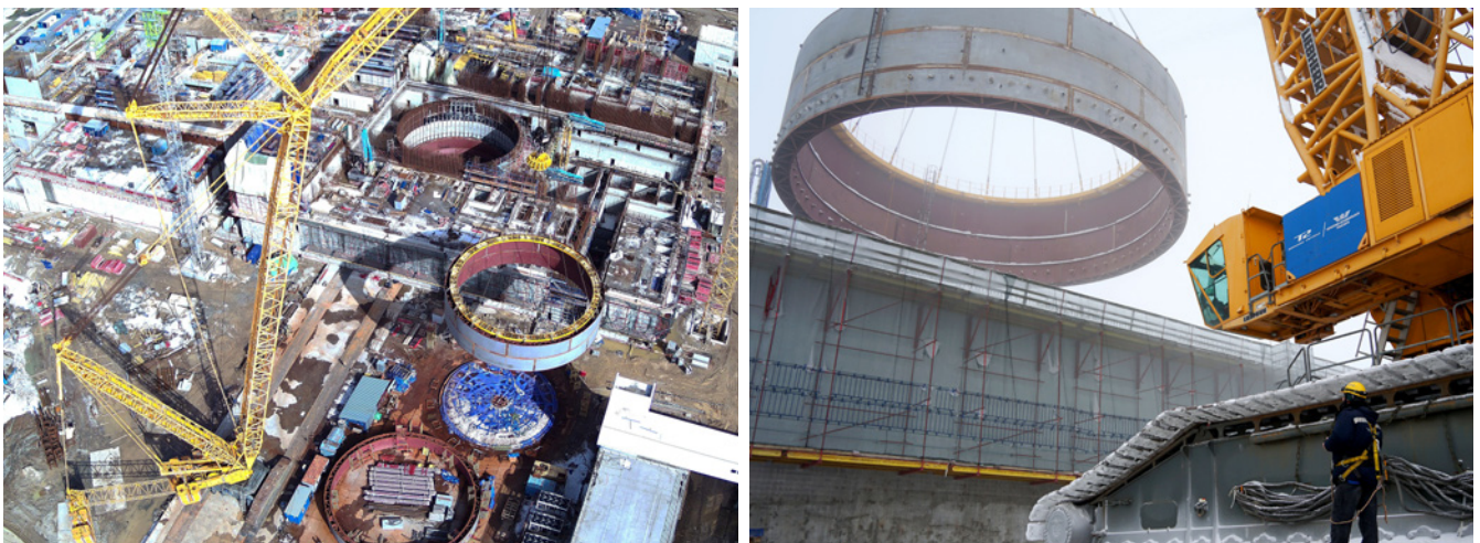
FIG. A.13. Construction status of BREST-OD-300 lead cooled fast reactor in Seversk, near Tomsk, Russian Federation, April 2024 (Source: Siberian Chemical Plant)
