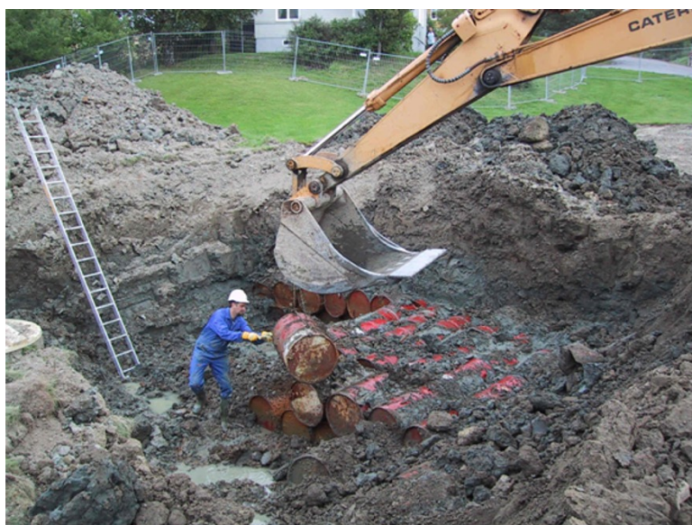
Retrieval of waste drums at the Kjeller site.
