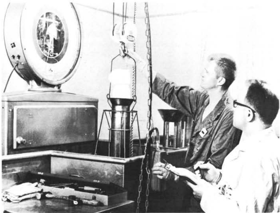
Plutonium from spent reactor fuel is weighed at the Nuclear Fuel Services Plant in New York and the details recorded by an Agency Safeguards inspector. The need to regulate the use of atomic energy for peace gives nuclear law its international and public aspect. Photo: USAEC
