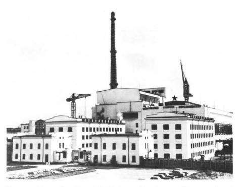
The power station at Novo Voronezh, USSR, has an electrical output of 210 megawatts and has been operating since 1963. It has a pressurized water reactor. USSR, whose first power reactor started operating in 1954, is now building a fast reactor at Shevchenko, described in this Bulletin.
