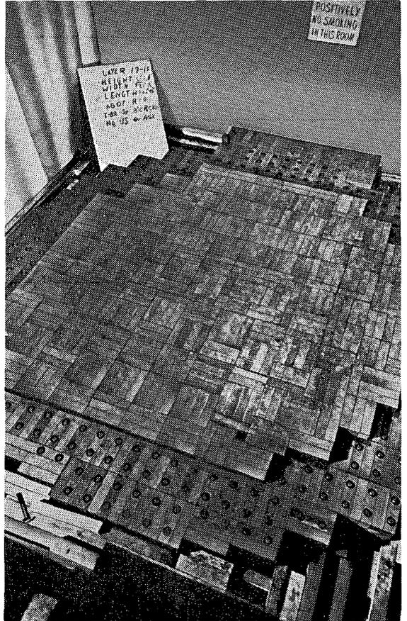
The only photograph of the world's first reactor during its construction at the University of Chicago. Taken in November 1942, it shows the basic design of the pile, with alternate layers of graphite containing uranium metal and uranium oxide, and spaced with layers of "dead" graphite... Argonne National Laboratory
