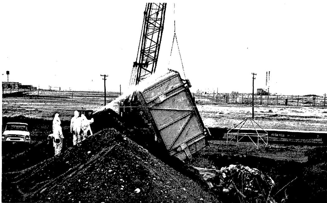
Rubbish which has low level radioactive contamination is loaded into a box, and dumped into a burial pit, at the Atomic Energy Commission's Hanford Works. It is being hosed to prevent possible spread of contamination by an errant breeze... Battelle-Northwest
