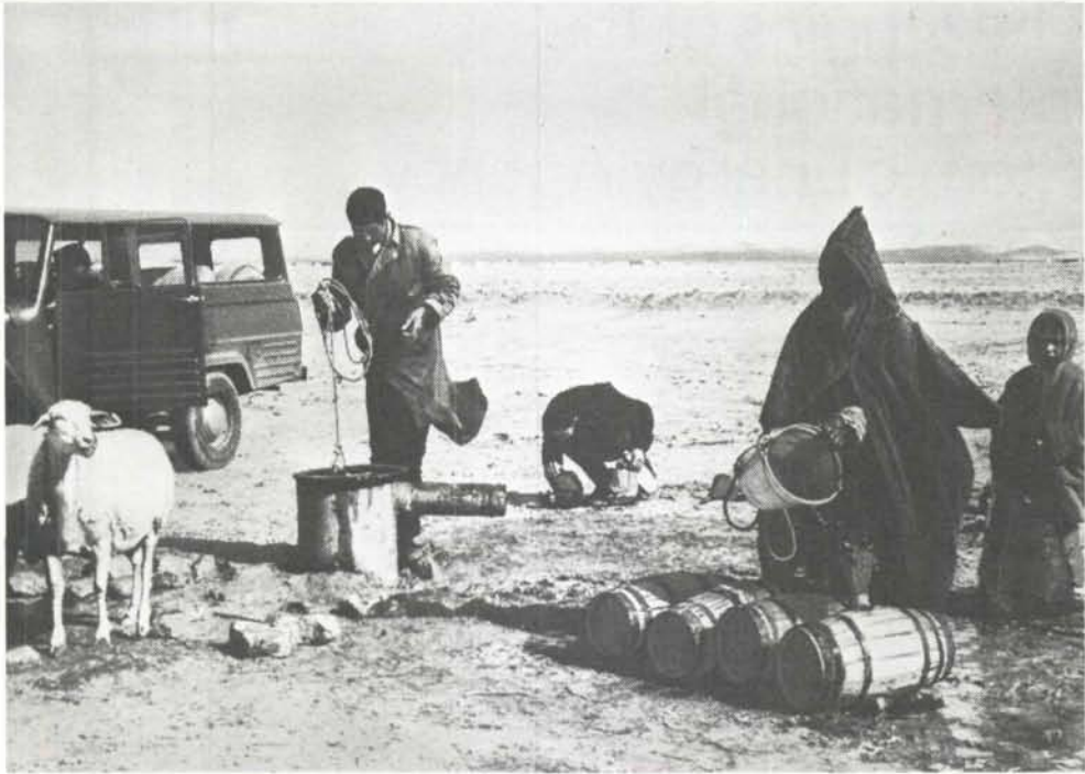
In the arid Hodna Basin area of Algeria water samples are taken from a well as part of an investigation of underground resources. Nearly 100 samples have been taken in a United Nations Development Programme plan executed by the Food and Agriculture Organization and assisted by the Agency.
