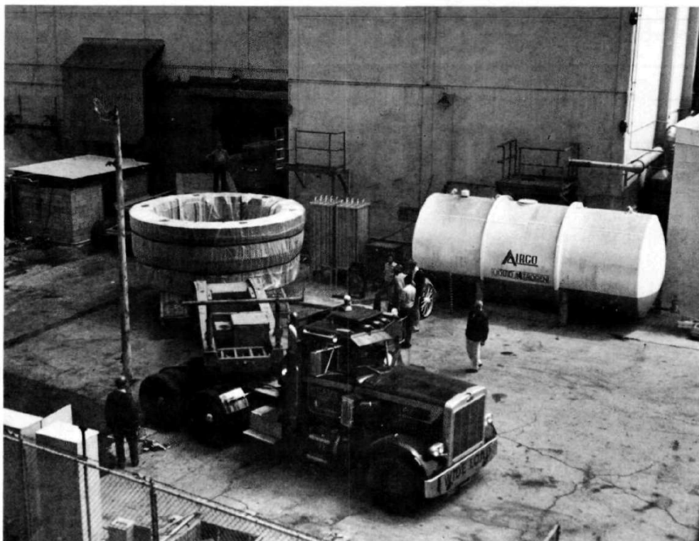
Part of the reactor from the SRE facility in California being shipped for burial. SRE was dismantled, with the job completed in 1982. (Credit: Rockwell International)
