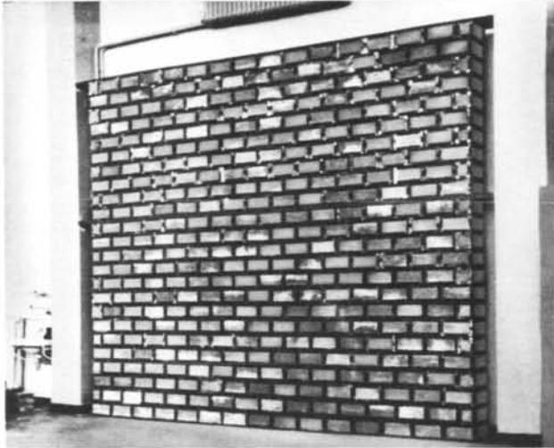
A wall of the reactor room at Vinca where the IAEA's dosimetry project was conducted. The wall is shielded by concrete bricks
