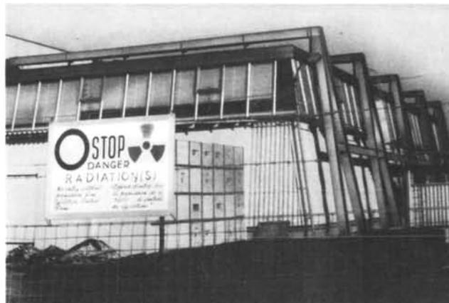
Cement blocks stored outside a cyclotron building for use as shielding against radiation
