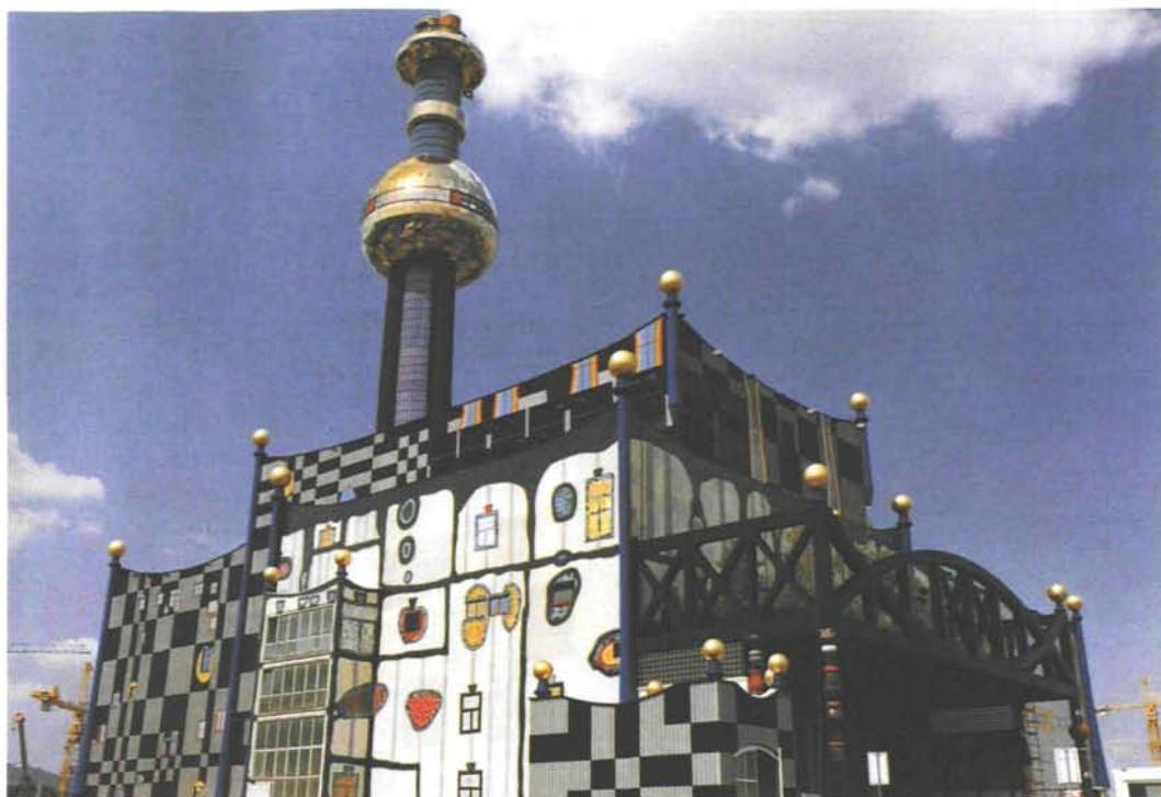
The municipal waste incineration plant in Vienna, whose facade was designed by Viennese painter, Friedensreich Hundertwasser. (Credit: E. Schauer, Vienna)
