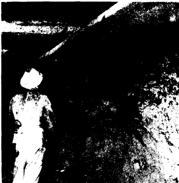
Polythene duct for ventilation of development headings (from paper by C.F. Smith)
