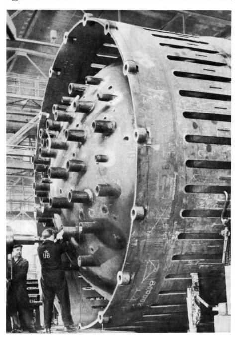
8 and 15 metres long respectively, of 76 mm molybdenum alloyed steel. lined with 5 mm stainless steel welded in ringe to the inner wall of the vessel. The two pieces will be held together by a new type of flange joint designed for the purpose by AB Atomenergie,
