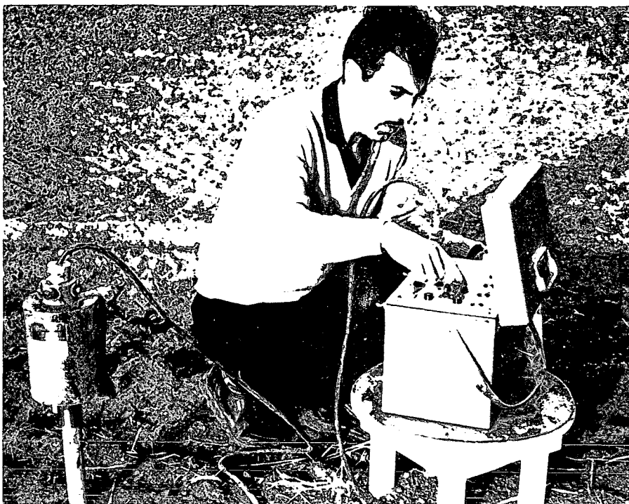
In research to find whether the old practice of allowing land to lie fallow each year is effective in conserving water measurements are being taken in Turkey using radioactive sources linked with instruments.
