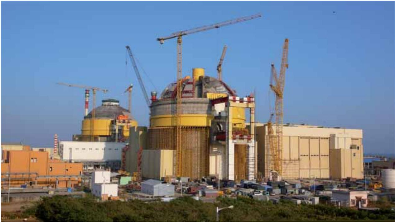
FIG. 1. Construction of water cooled reactors ( $2 \times 917$  MW(e)) at Kundankulam, in India.
