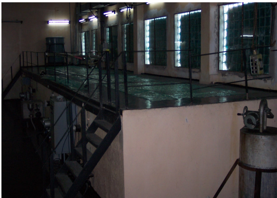
Spent fuel storage pools at the VVR - S Reactor of IFIN-HH
