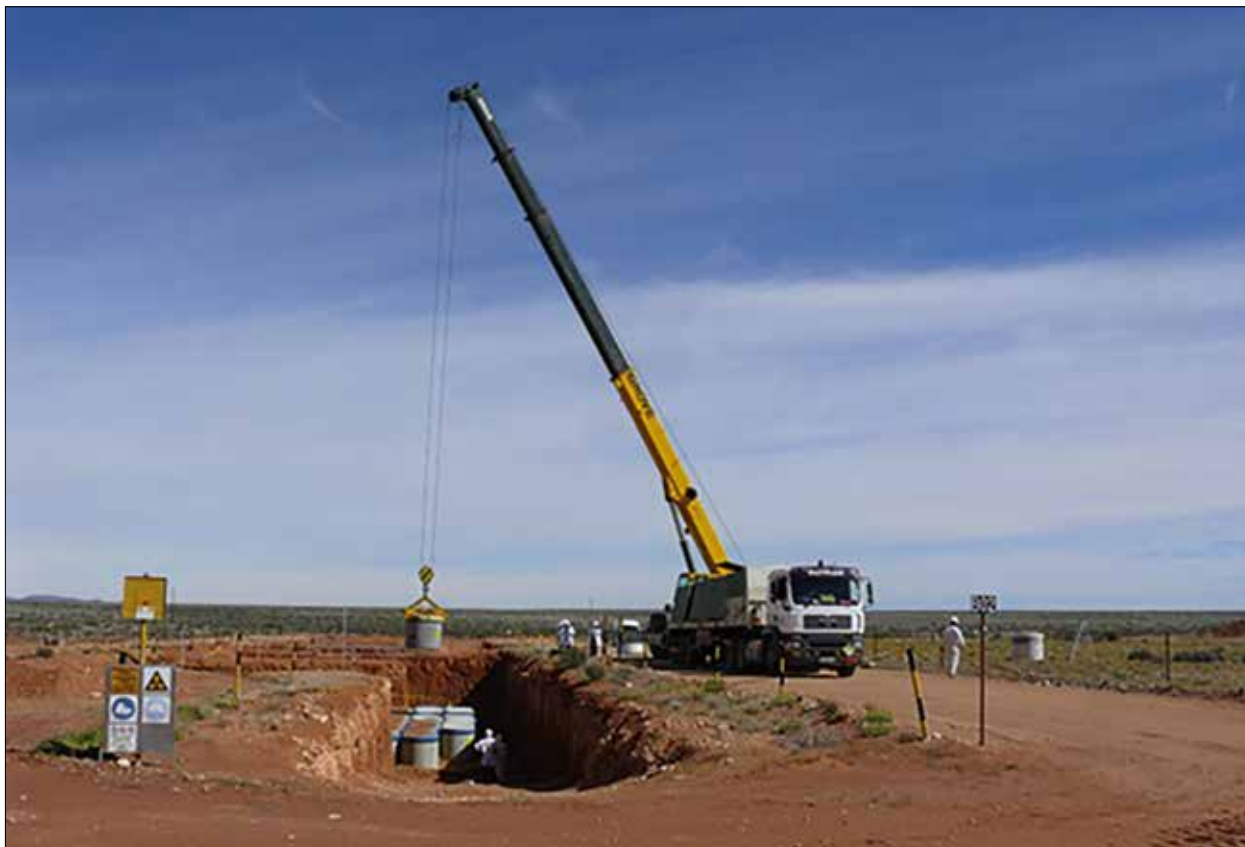
Figure 23: Concrete waste packages being placed into a disposal trench
