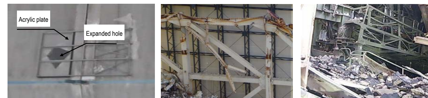
Figure 9: Upper part of Unit 1 Reactor Building – Covering status of hole in roof panel and status of rubble investigations
