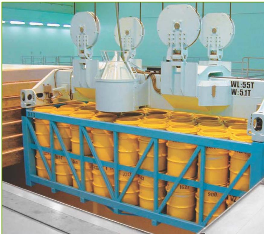
Figure 10: Storage of low-level operational waste in ZZL (Photo: Zwiilag)
