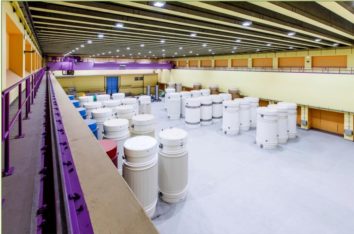
Figure 8: Transport and storage casks in the hall for dry storage at the Central Interim Storage Facility ZZL (Photo: Zwiilag)
